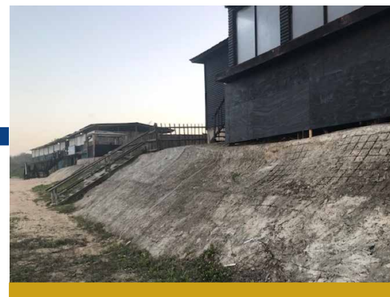
Right: Sea defence structures on coastal properties at Ponto d'Ouro. Erosion within the bay at Ponto d'Ouro has become more prolific as development encircles it and an equilibrium shift in the sand sharing system arises because of the closure of the sand bypass to the south.
